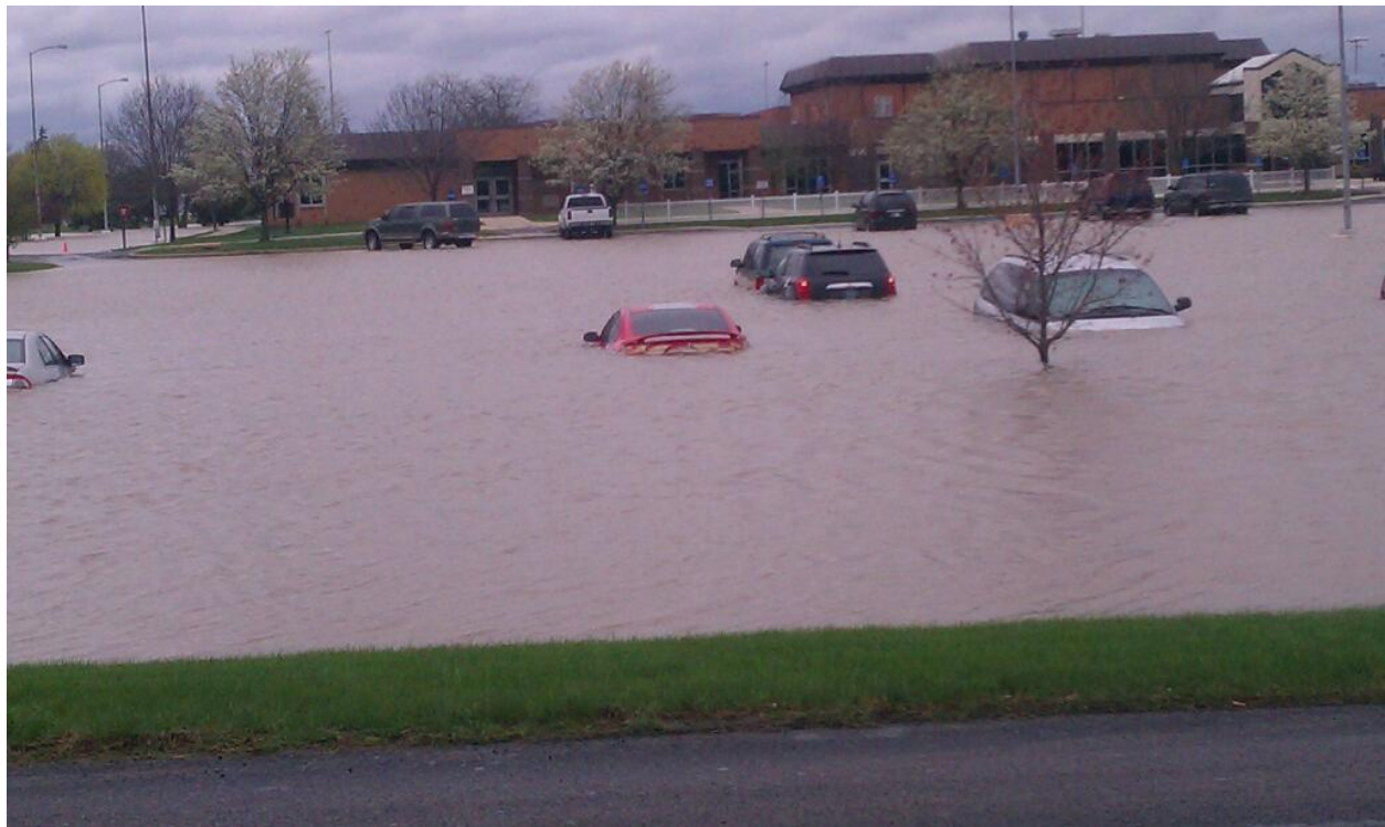
Figure 3: Flooding at Tipton Elementary School, April 2013
