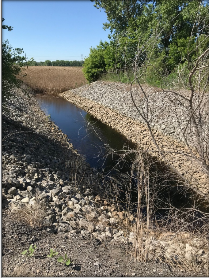
Photo 11: Proposed Location of Control Structure at Heron Rookery, Looking Upstream
