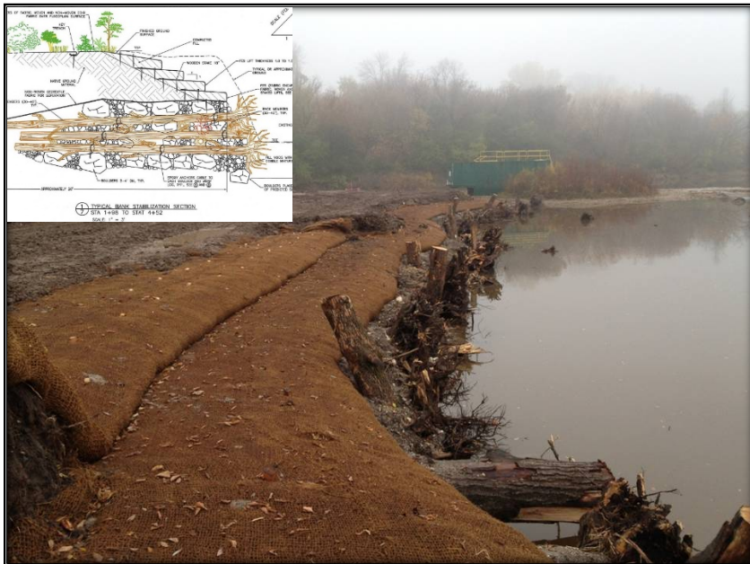
Photo 6: Large Woody Debris Structure and Soil Terracing, AER
