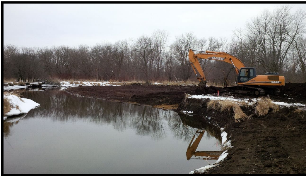
Photo 3: Grading River Bank to Mimic Natural Slopes and Morphology at Nippersink Creek, AER
