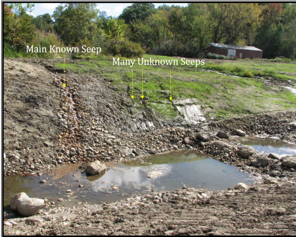
Photo 10: Adaptive Management of Seeps 1 st and 2 nd Year of Construction Red Mill Pond AER
