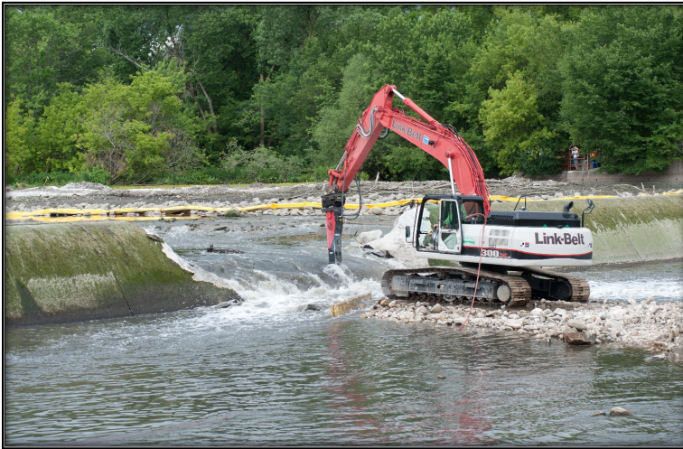
Photo 1: Demolition of the Hofmann Dam, Aquatic Ecosystem Restoration (AER)
