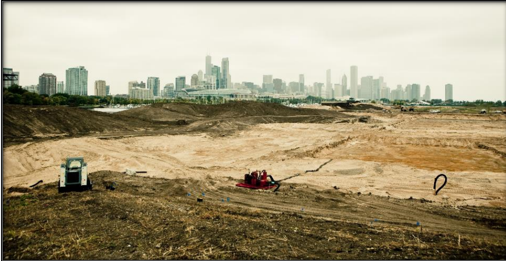
Photo 2: Excavation of Lacustrary Lagoon at Northerly Island, AER
