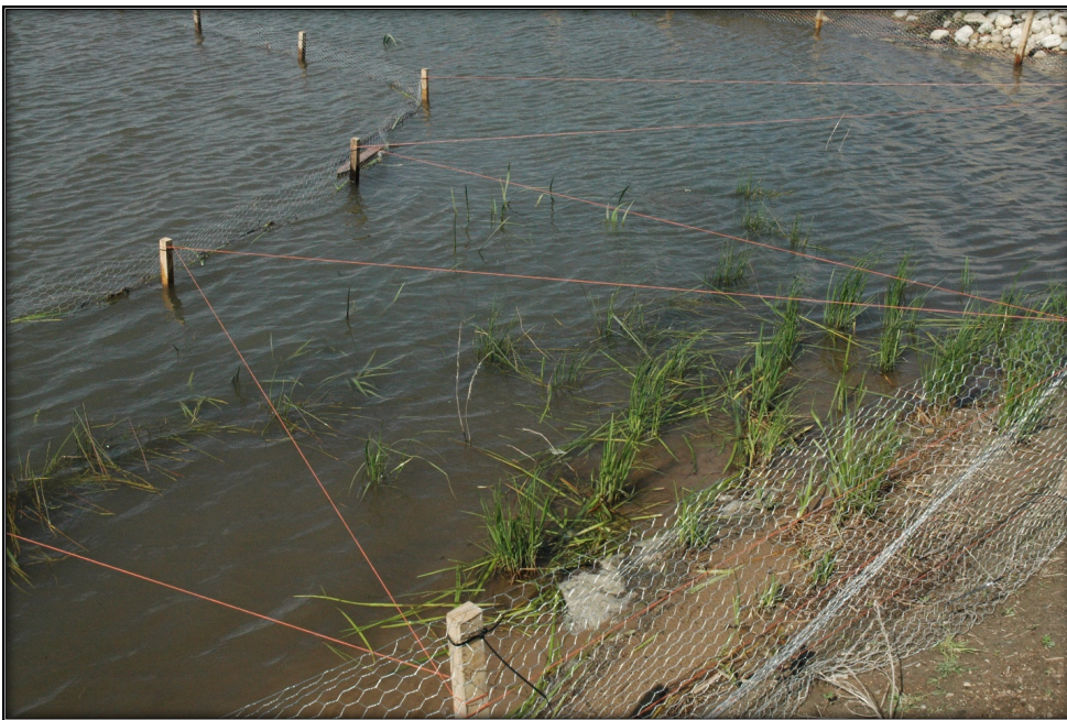
Photo 9: Common Carp and Canada Geese Protection for Newly Planted Wetlands Plugs, AER
