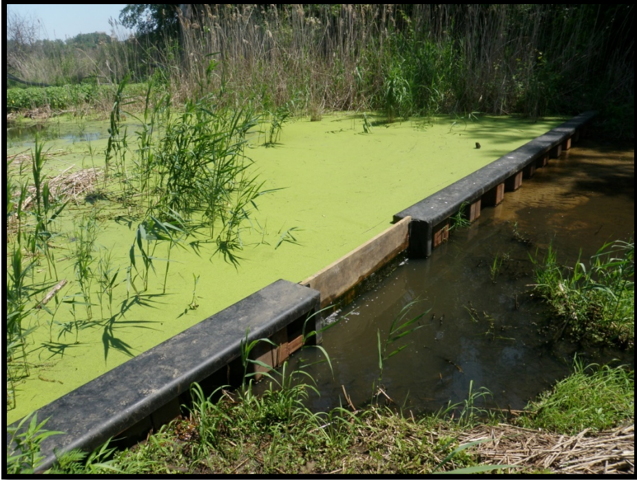
Photo 4 Water Control Structure to Stabilize Hydroperiod at Indian Ridge Marsh, AER
