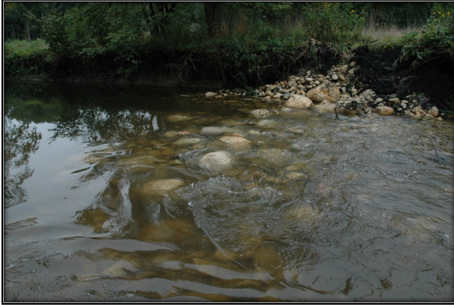
Photo 5: Boulder & Cobble Riffle Placement East Branch DuPage River Morton Arboretum, AER
